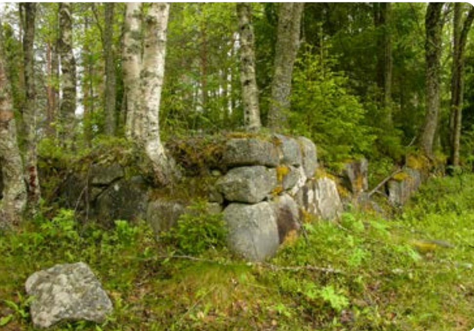
The birch trees that grow on the stone walls have caused the stones in the foreground to collapse. Most trees that are located in cultural heritage sites should be removed. Mickelstråsk, Västerbotten.
